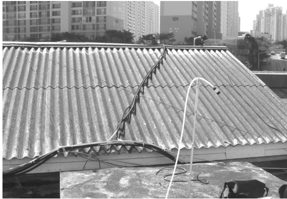
a) The roof of a plant
