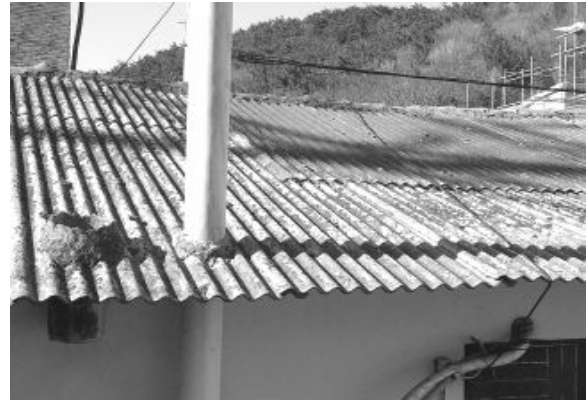
b) The roof of a residential house
