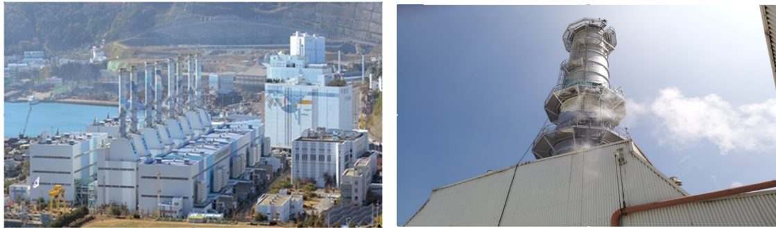
Fig. 2. Korea Southern Power CO., LTD(BUSAN) & the foreground of unit 8.
